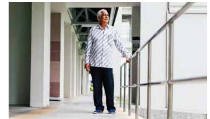
Void deck aprons which have been levelled, with additional handrails for support.
