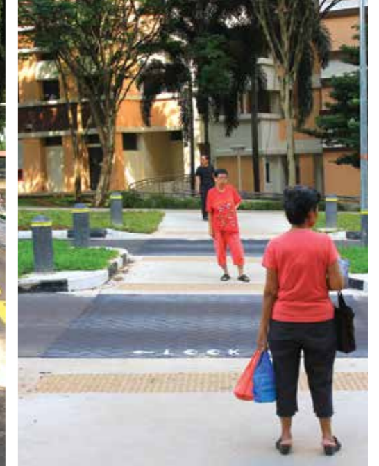
(Above) 'LOOK' markings painted at road side ramps to remind pedestrians to look out for traffic. A special pedestrian refuge is also installed in the middle of the road for pedestrians to cross the road safely in two stages. Tactile tiles enable visually-disabled persons to better navigate the roads safely.
